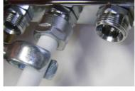
Manually screw the nut to the connection and tighten it by using an open polygonal wrench for hexagon 27
