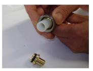
Insert the nut with pre-assembled retaining ring on the pipe to connect
