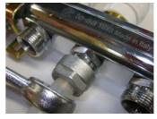
Manually screw the nut to the connection and tighten it by using an open polygonal wrench for hexagon 27 mm
